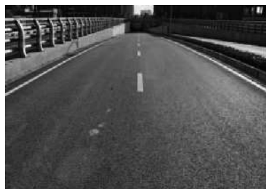
Xiaying Avenue, Ningbo
